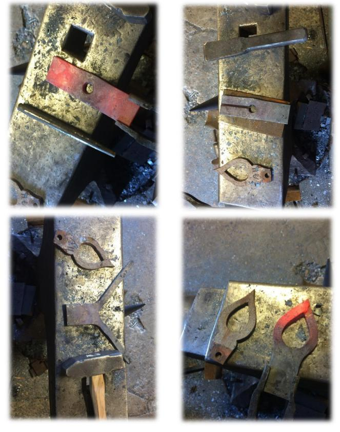
Our next step was to replace some of the forged elements that were either missing or too damaged to be restored. Above are a series of photos that illustrate the various traditional blacksmithing techniques and tools that were necessary to make some of the pieces.
