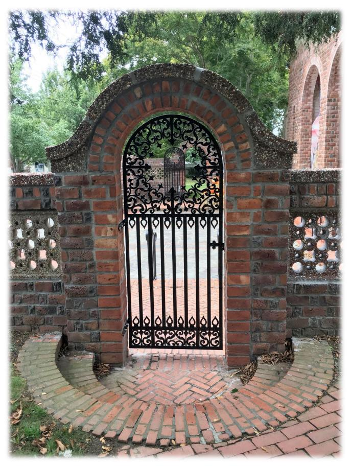
Here are the restored gates re-installed in their original locations complete with a new latches, custom hinges, metalized and painted finish. They are now ready to withstand years of service.
