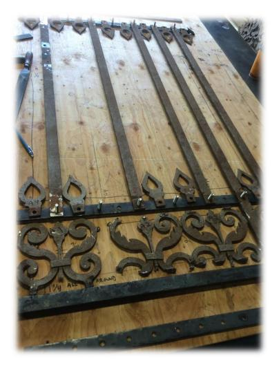
Once assessed, the gates were then completely disassembled. During this process, we found that all of the metal components within the gates were held together with mechanical connections. The majority of these connections were riveted together so each rivet had to be drilled out individually.
