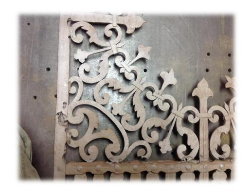
After closely assessing the gates, we found that the frames, crossbars, and some of the infill were badly rusted and required either extensive repair or in some cases, complete replacement in certain areas. Here, you can see an overview of the rust, wear and damage.
