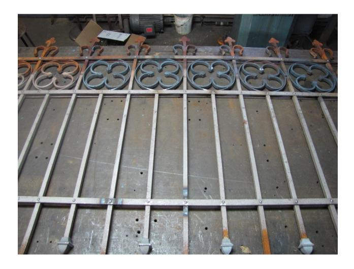
Once the parts were straightened, they were placed on the layout table and reassembled. Bolts were used to as stand-ins for the rivets during this part of the process. One by one, the bolts were removed and new steel rivets were installed into the existing holes. They were then hammered down while hot with a cup shaped tool to form a new head. As the rivets cooled, they shrunk and formed tight solid joints that created a water tight seam when painted.
