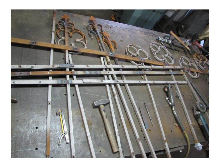
Once the ironwork was uninstalled, it was transported back to our yard for dismantling. The severely damaged sections were sent out and sandblasted to remove the old paint. This was done so our workers could see the full extent of the damage and work with clean material free of paint that would not produce harmful fumes when heated. We then removed all of the pins, rivets and bars. The bars were then separated and straightened by hand.
