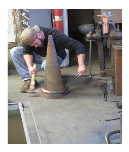
The fencing contained many quatrefoil rings that were crushed. In order to return them to their original shape they were heated and dropped over a cone mandrel. The smith then carefully hammered the ring back to round. Bolts were used to hold all of the parts in place prior to riveting.
