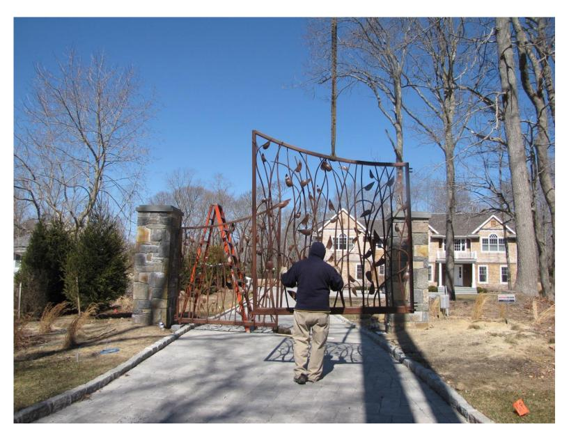
The gates were delivered to site via the company truck and lifted into place using a crane. This was necessary due to the weight and size of the gates. The gates were then bolted in place using an adjustable hinge system. This allowed for the gates to be adjusted so that they line up perfectly and if ever necessary, any misalignment that may develop could be easily corrected.
